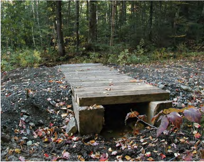
Wood Box culvert: no gravel cover needed
