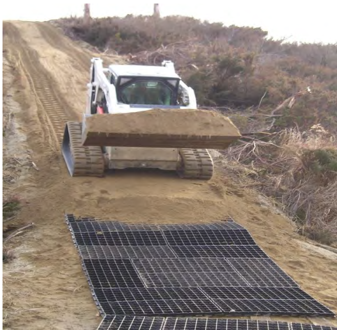
Geoblocks are best used to harden wet sections of trail.
